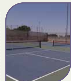
Installed the Ray Kroc pickleball courts
