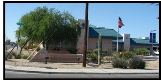
City of Yuma Public Works Department
