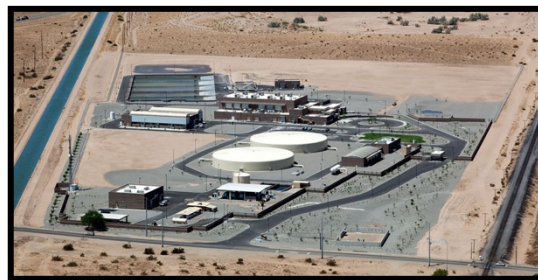
Agua Viva Water Treatment Facility
