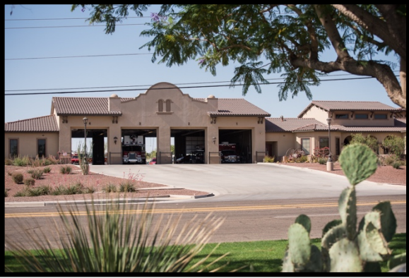
City of Yuma Fire Station No. 1
