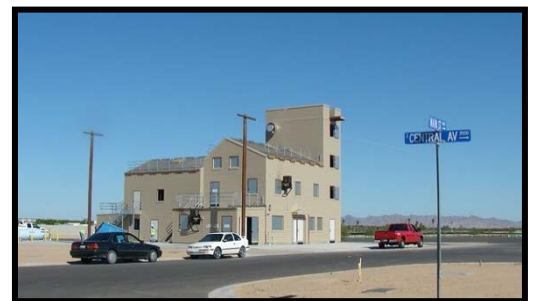
Burn Building located at the City of Yuma Public Safety Training Facility
