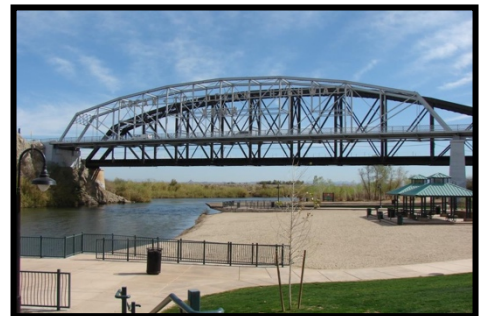
Ocean to Ocean Bridge over the Colorado River.
