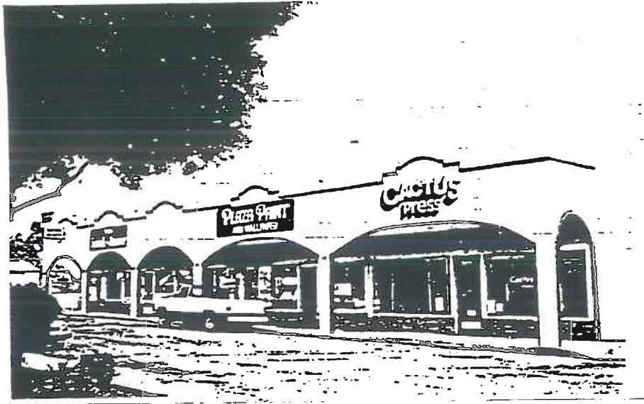
CACTUS PRESS/PLAZA PAINT BUILDING YUMA MRA
