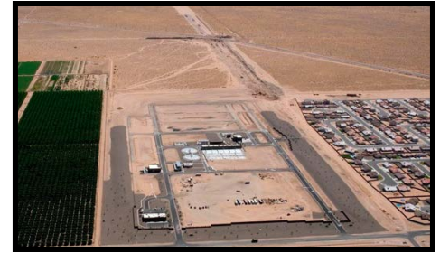
Desert Dunes Water Reclamation Facility
