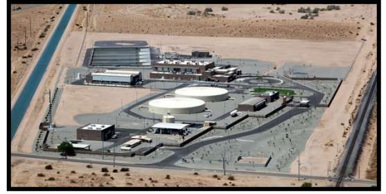
Agua Viva Water Treatment Facility
