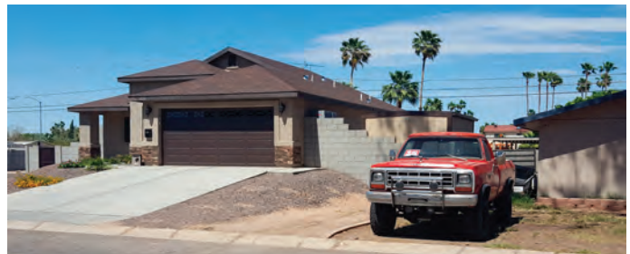
Home built on several feet of fill to raise it above the flood level.
