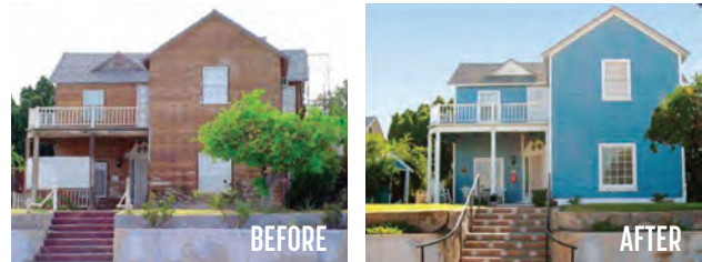
YCNHA's facade restoration program helped revive this home on Orange Ave.
